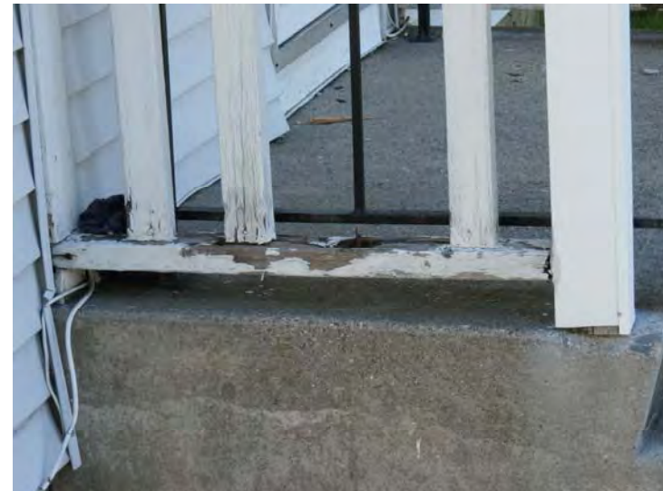
Example of porch deterioration
